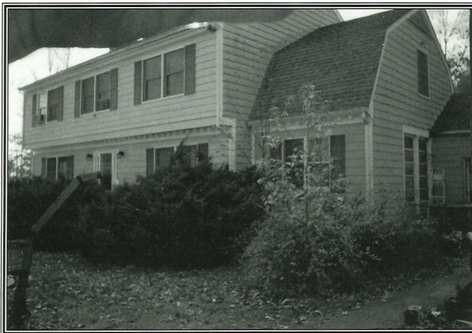
That's the kennel between the garage and the main part of the house. And, yes, that's John's hand at the top.
