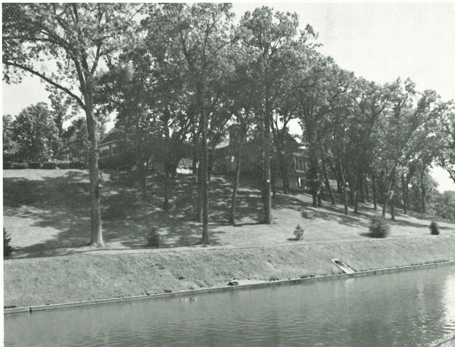
Rear view of main house at Knolland Farm
