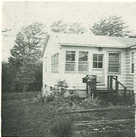
This is the addition Betty and Rex added two years ago. The front room is a show-room, and in the back is the nursery.
