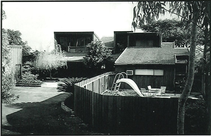
The front view of the Hattori dwelling
